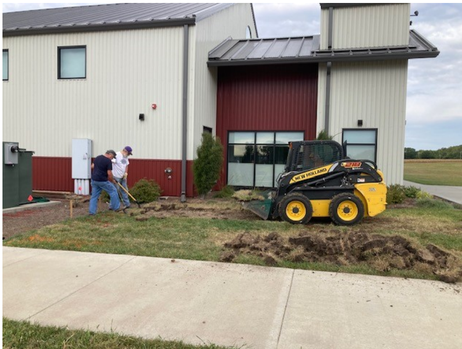
Skimming off the top soil to be saved.
